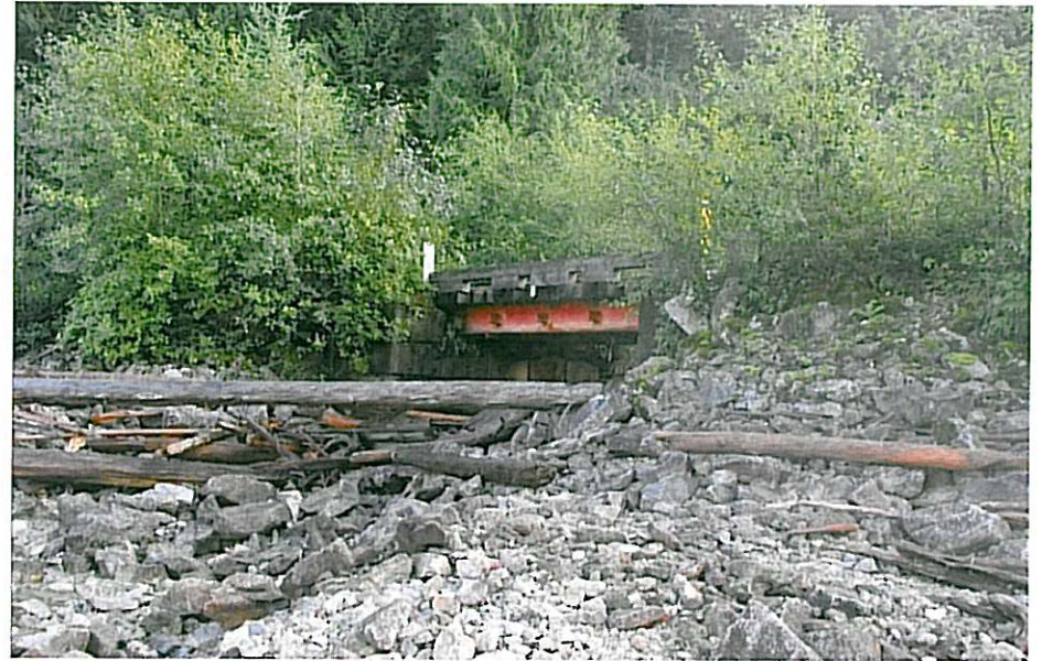
CK-2327 From downstream
